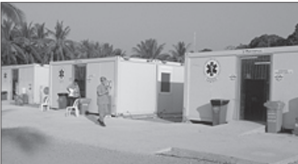
Fig 6: Temporary mortuary consisting of three buildings
