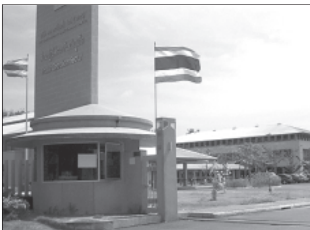
Fig 11: Thailand Tsunami Victim Identification Information Management Centre
